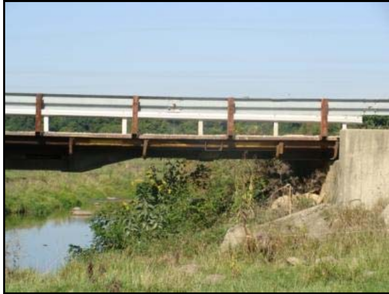
Figure 3.17: RRFC bridge supported outside of wheel truck
