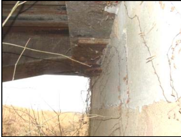
Figure 3.16: Integral abutment on RRFC bridge
