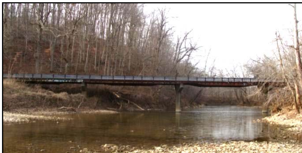
Figure 3.19: Four span RRFC bridge
