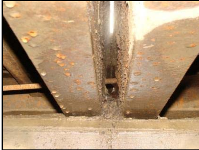
Figure 3.12: Threaded rod longitudinal connection
