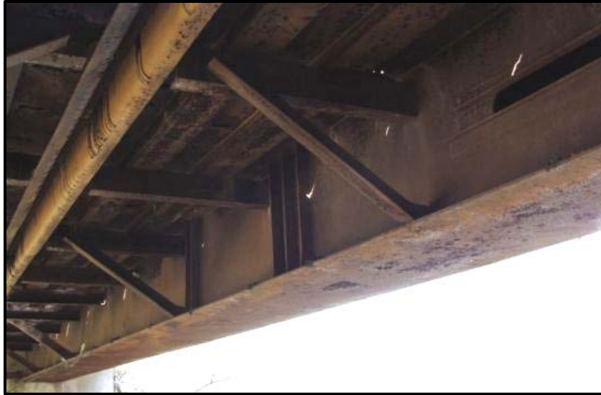
Figure 3.3: Typical box girder
