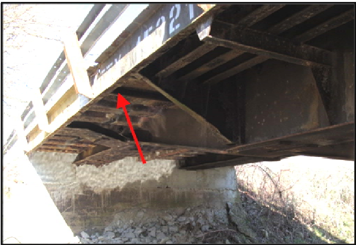
Figure 3.5: Typical channel exterior girder
