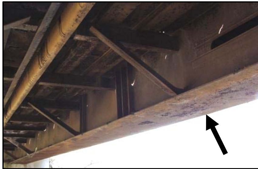
Photograph of typical main box girder
