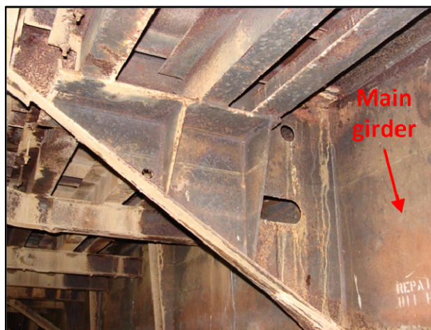
Figure 3.9: Typical large transverse member
