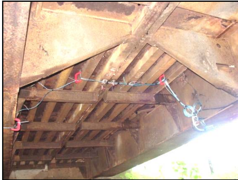
Figure 4.2: General view of strain gages installed at midspan of CL-53
