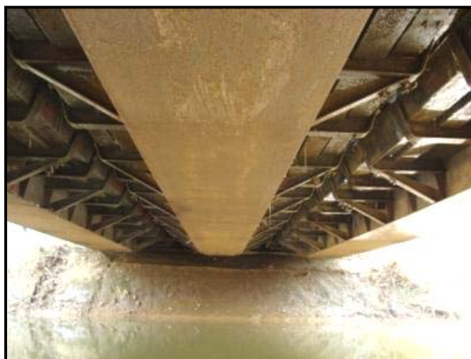
Figure 3.11: Bridge constructed of 3 RRFCs side-by-side
