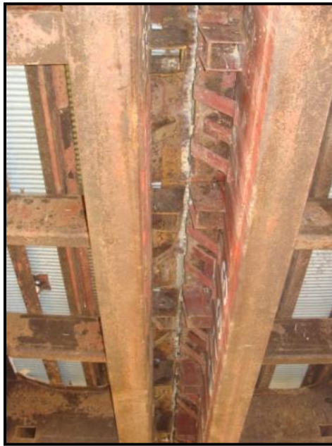
Figure 3.14: No connection between RRFCs
